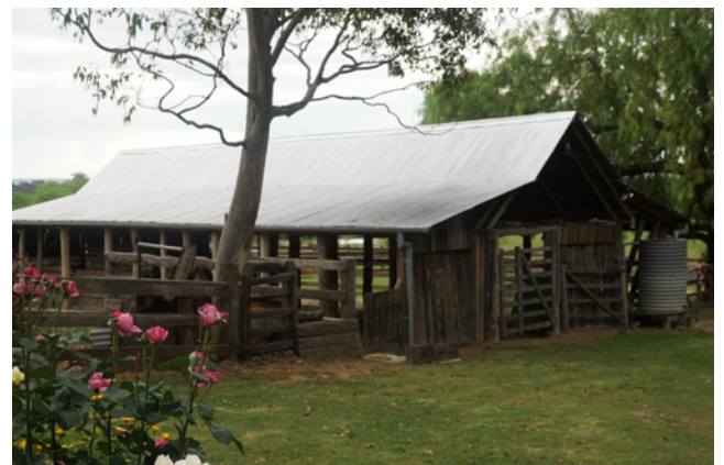
Barn after restoration
