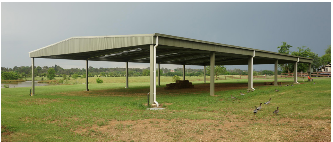
New Building - Covered Outdoor Working Area (COWA)
