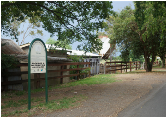
View of fencing across dairy building yards area
