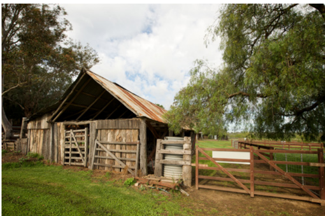
Barn before restoration
